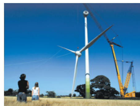
An Ecotricity turbine being erected.
